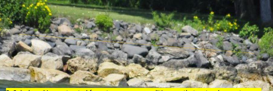
3. Splash pad is constructed for extreme wave conditions so that water does not come over the armor stone and erode the bank behind the revetment
